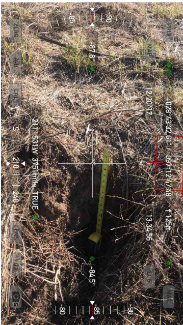
9718 - Exterior Erosion, Possible Borrow Near Toe
