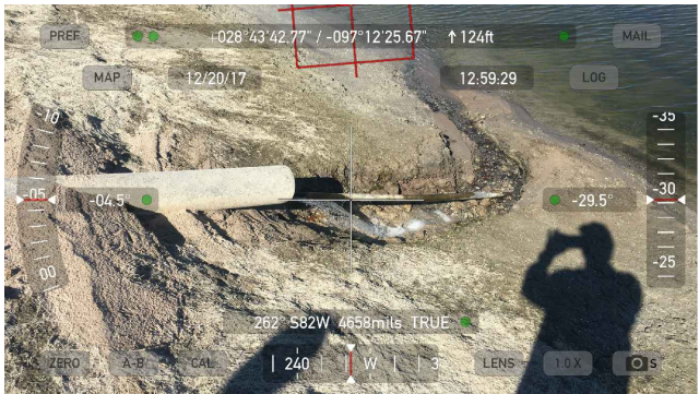
9659 - Discharge from Primary Ash Pond to Secondary Pond
