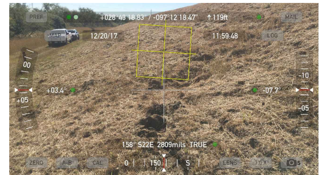
9551 - Exterior, Hog Damage
