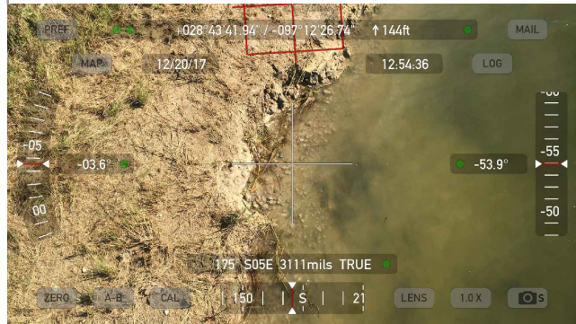
9645 - North Dike Interior, Erosion Below Slope Armor
