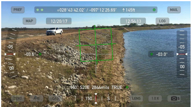
9644 - North Dike Interior, Erosion Below Slope Armor
